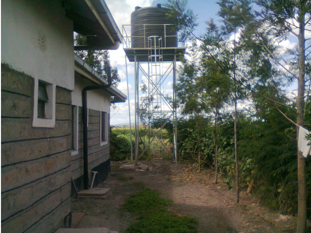
The tank and the tower which pumps water in the house.
